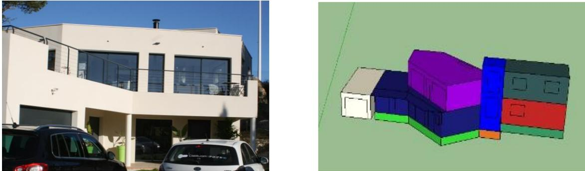
Figure 1: Outside view of the building, EnergyPlus model.
