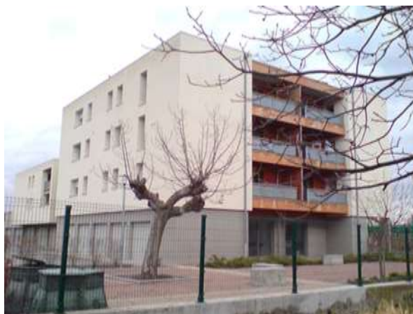
Figure 1 : Exterior view of the base case study
