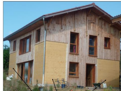
Rammed earth walls
